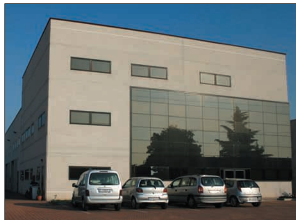
INTEK S.R.L. Head Office & Logistics Building Segrate - Italy
